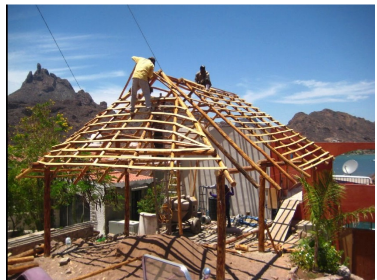
These men are preparing a frame, which will be topped with woven palm branches to form a palapa
